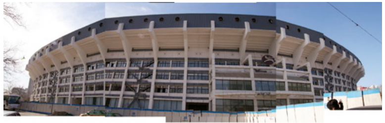
STADIUM UNDER RECONSTRUCTION
